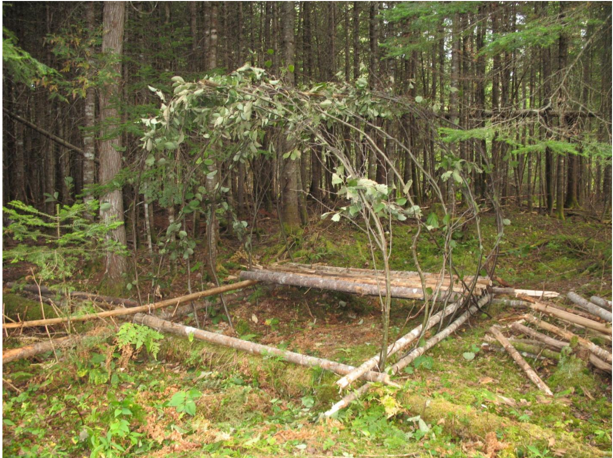
Figure 4. Large Hoop House Frame With Alder Rafters. This picture shows the completed frame, bed (without the bough mattress), and the alder saplings twisted together to form the arched rafters.
